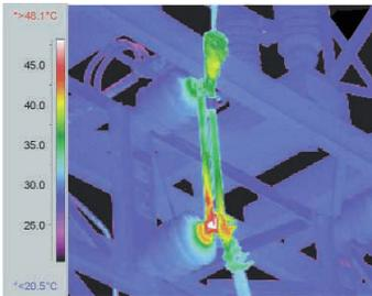
The white areas shown here indicate overheating on one of the fingers of this disconnect switch.
